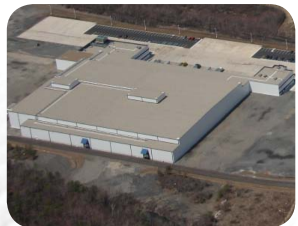
U.S Cold Storage is one of several national cold chain companies that provide space in NEPA.
