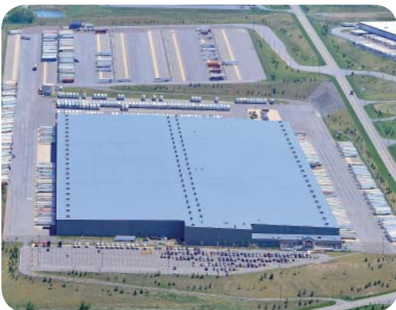
Lowe's distributes its products from a 1,582,112 square foot, 700+ employee NEPA facility.
