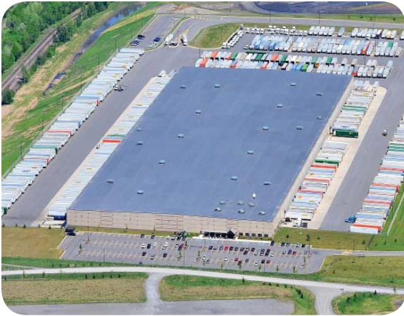
The Home Depot operates a 465,600 square foot, 350-employee regional distribution center building in NEPA.
